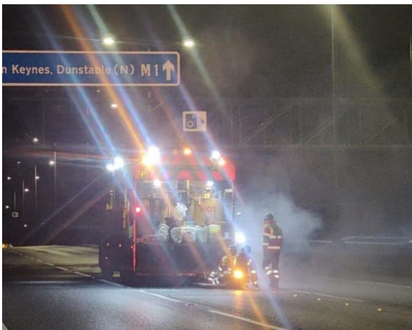
Installing temporary road studs (cat's eyes)
