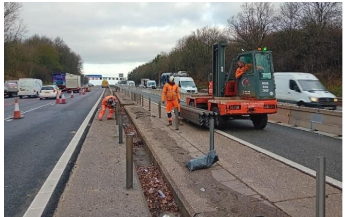
Removing the existing steel central reservation barrier
