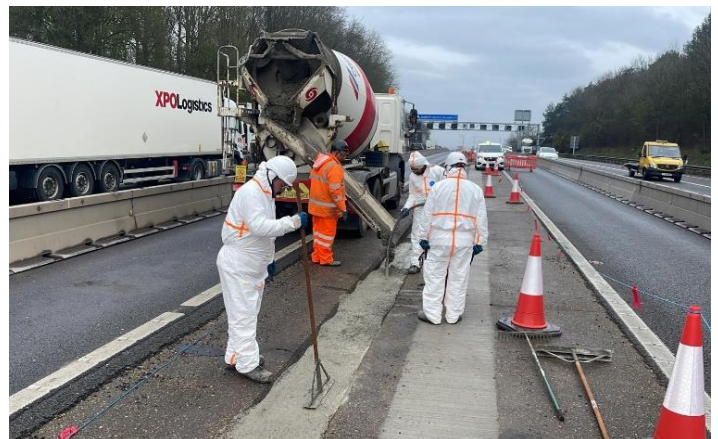
Concrete infilling
