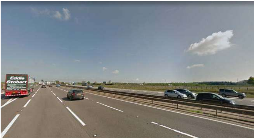
4-view from M1 looking north with site to the right
